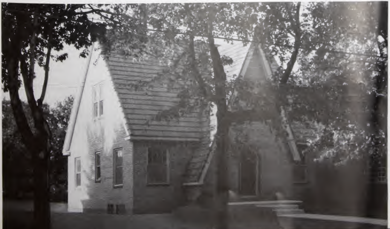
Buff mat glazed Dunbrik home with a green mat glazed Duntex roof, Metropolis, Illinois.
